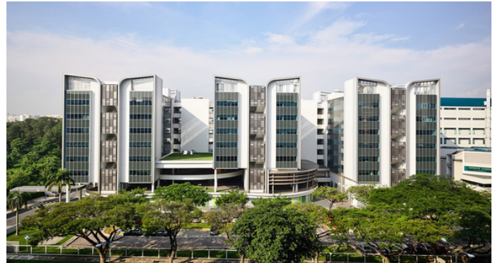
Temasek Polytechnic East Wing Block 1A
